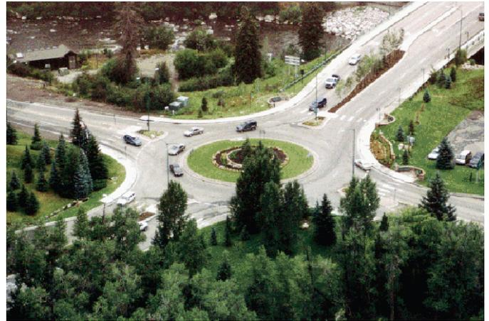
built. Roundabouts are not the best solution in every situation. In the case of the Northwestern Connector Project, it was found that the proposed roundabouts will provide a level of service above that which could be obtained by convention signalized intersections while providing the excellent safety features previously mentioned.
